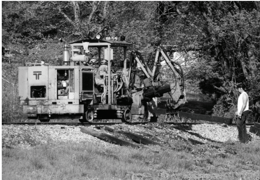
The Fredonia Valley Railway (Princeton to Fredonia, KY) gets some new ties as the line is upgraded in April 2007. Photos by Bill Thomas (film/scan)
