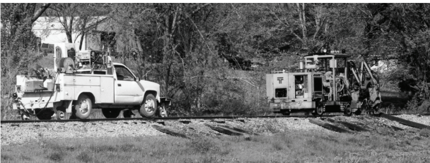
The Fredonia Valley Railway (Princeton to Fredonia, KY) gets some new ties as the line is upgraded in April 2007. Photos by Bill Thomas (film/scan)
